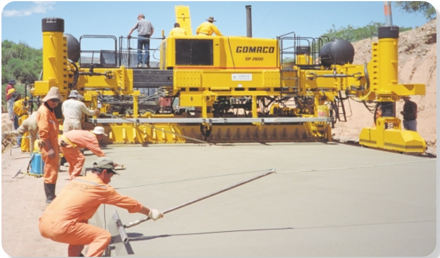
This versatile four-track GP-2600 slipforms a 24 ft. (7.32 m) wide concrete roadway near Cochabamba, Bolivia.
