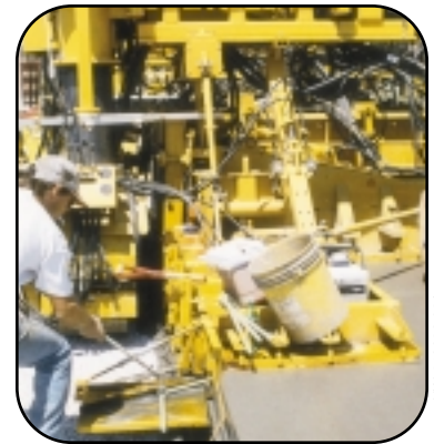
Trailing Form With Manual L-Bar Insertion
