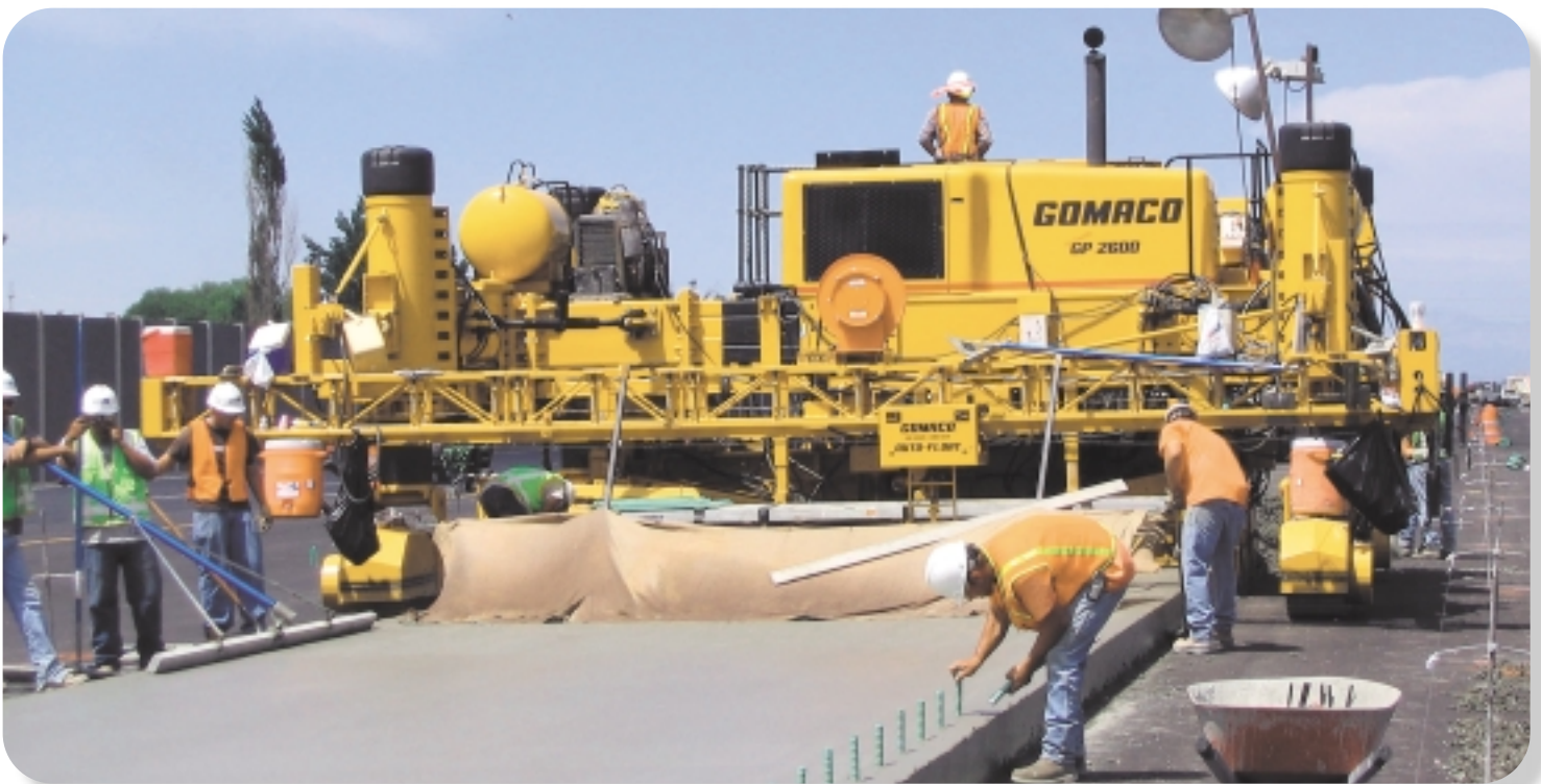
This versatile four-track GP-2600, equipped with the GOMACO Auto-Float® slipforms mainline paving in Salt Lake City, UT.
